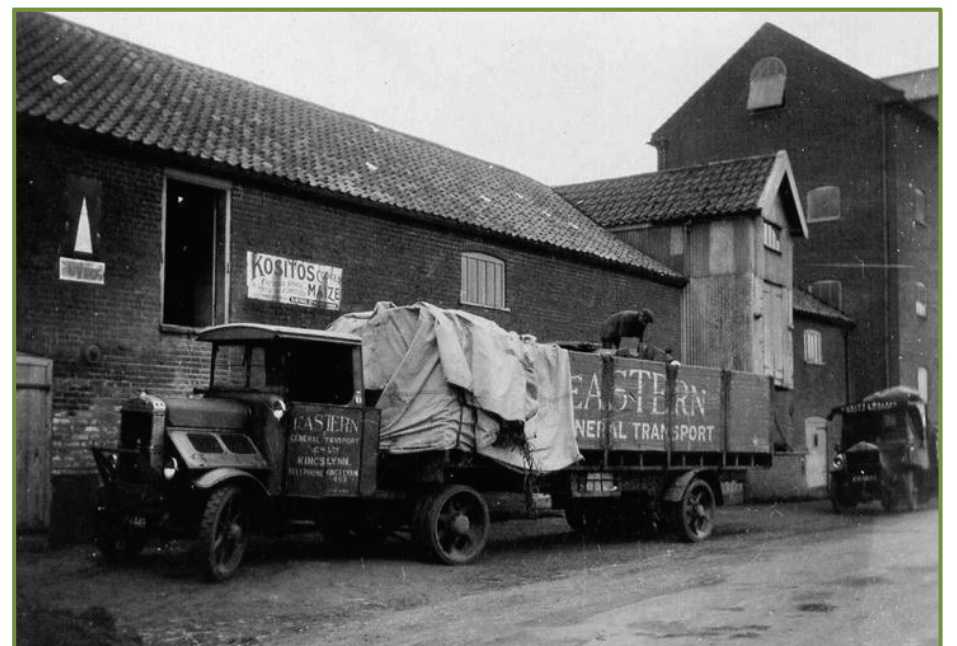
Loading sacks outside Ebridge Mill, c1920s
